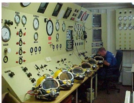
PDC FIRST SATURATION DIVE PANEL NOW LOCATED IN CLASSROOM AS AN A/ LST TRAINING PANEL
